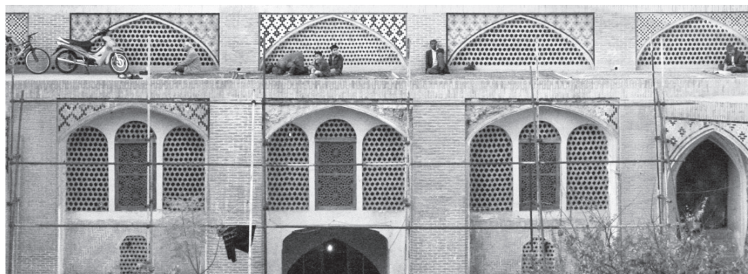
▲ Figure 2. Stone latticework windows in Aqa-Bozorg mosque-school.
