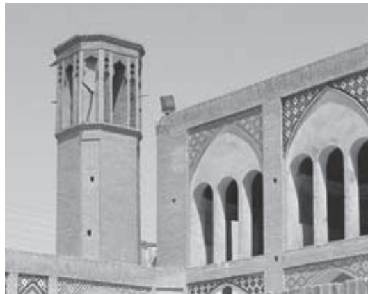
▲ Figure 4. Element of airflow variability (Bad-Gir) in Aqa-Bozorg mosque-school
