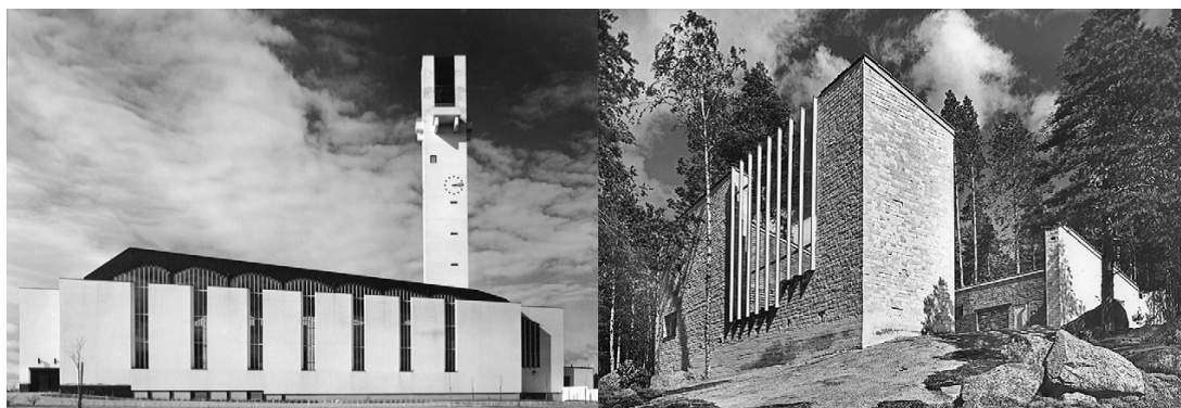
▲ Figure 1. Church of the Plains by Aalto, 1951–1960. Note: Photo: Kalevi A.M'äkinen, Alvar Aalto Museum. Approximately 1960. & Figure 2. Muuratsalo, Experiment alHouse by Aalto, 1952– 1954. Note: Photo: EinoM'ökinen, Alvar Aalto Museum.
