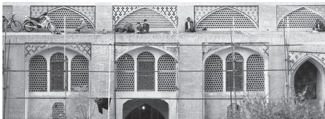
▲ Figure 2. Stone latticework windows in Aqa-Bozorg mosque-school.
